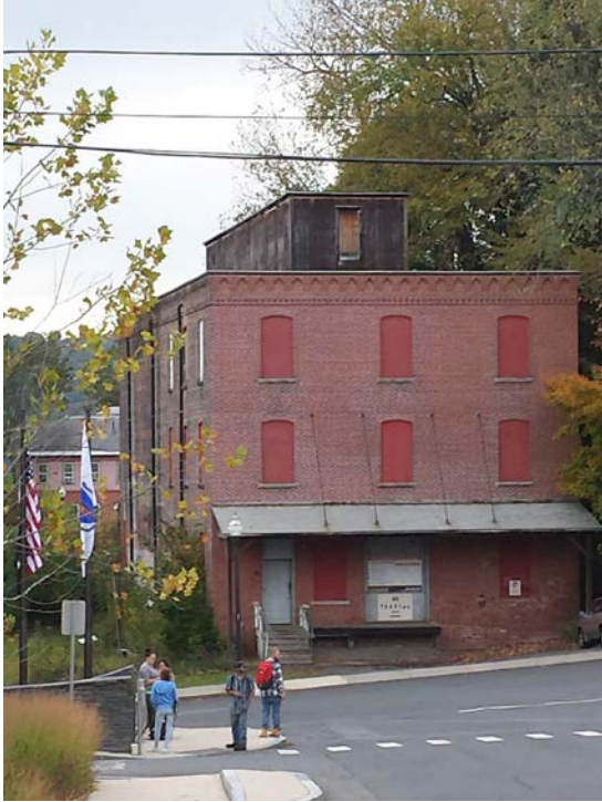
Figure 12: Existing front (East) facade
