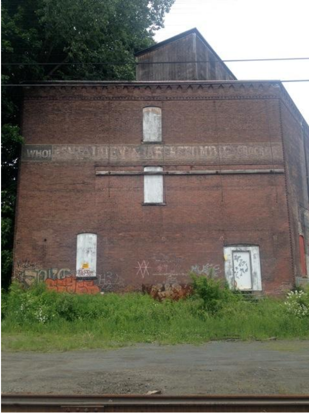
Figure 14: The West facade
